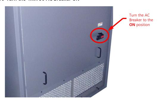
Figure 17 – Turn the 4MX 50 AC Breaker to ON
