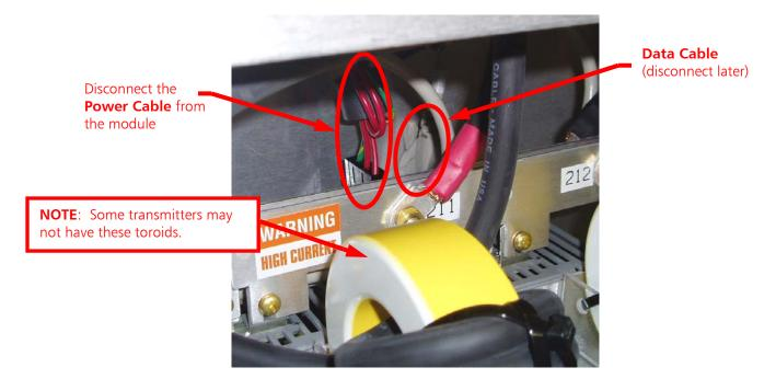
Figure 4 – Disconnect Power Cable
