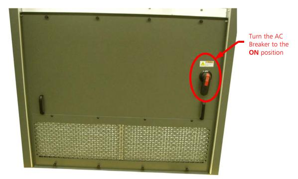
Figure 14 – Turn the AC Breaker to ON
