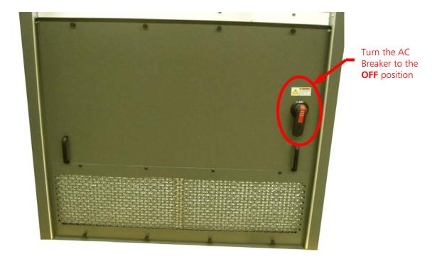
Figure 1 – Turn AC Breaker to OFF
