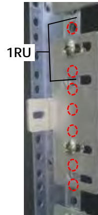
Figure 6 – Right Rear Support Mounting
