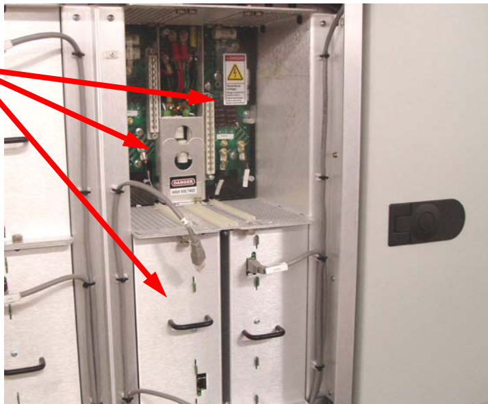
Figure 166 – Install PA Modules
