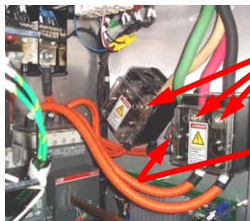
Figure 130 – AC Terminal Block Connections
