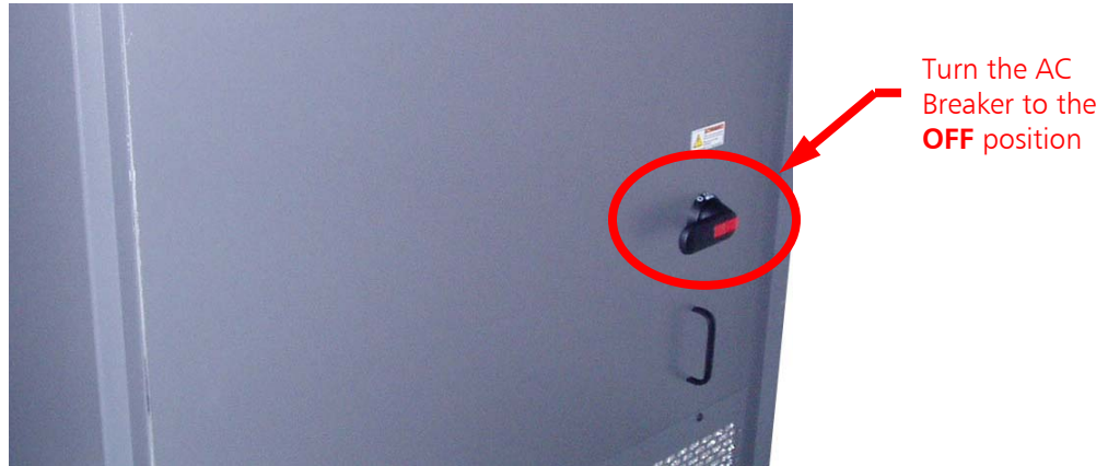
Figure 210 – Turn 4MX AC Breaker to OFF
