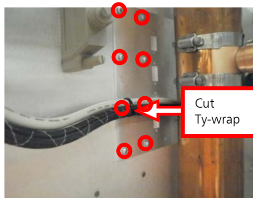
Figure 48 – Remove Existing Panel
