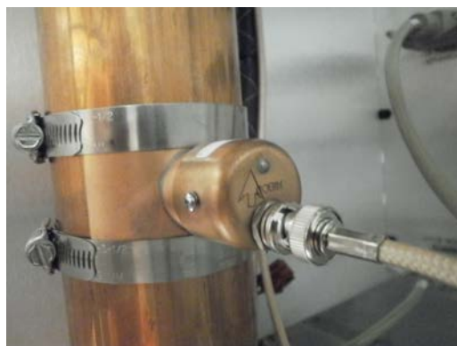
Figure 47 – 3 1/8" Coupler Installed
